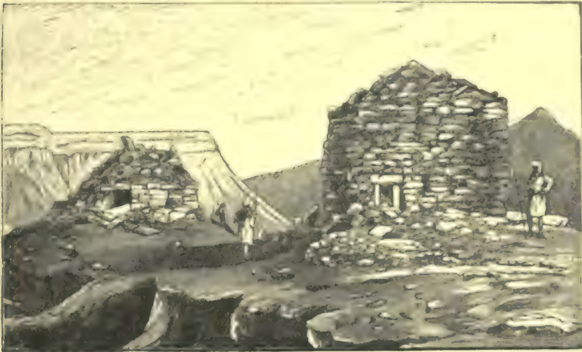
TWO REFUGE TOWERS OF THE HIRŪ-SHĀĪTŪ, IN THE WADY BĪAR. 1
